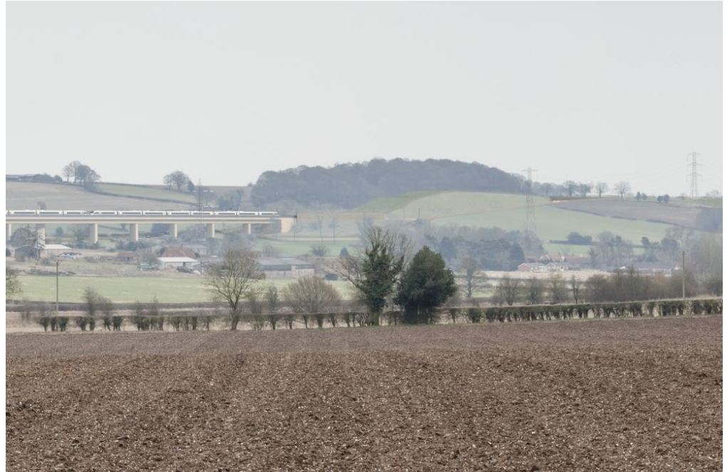
Wendover Dean viaduct: worst visual impact along route
